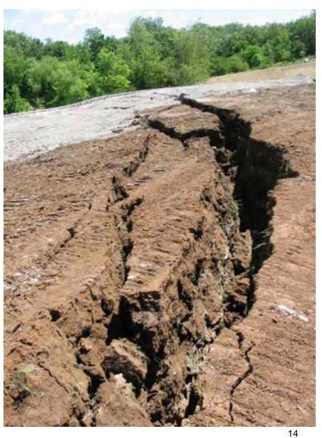
Tension cracks behind top of wall
